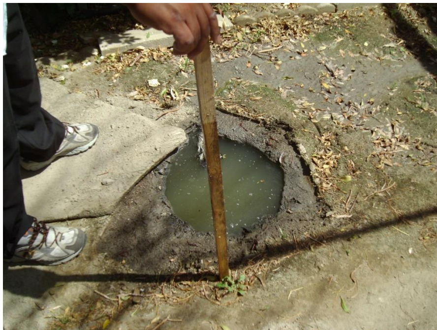
Example of Surfacing Wastewater from an Undersized Septic System
